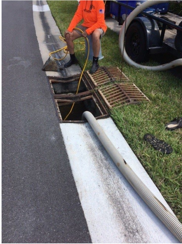
SWM - Drainage Structure
