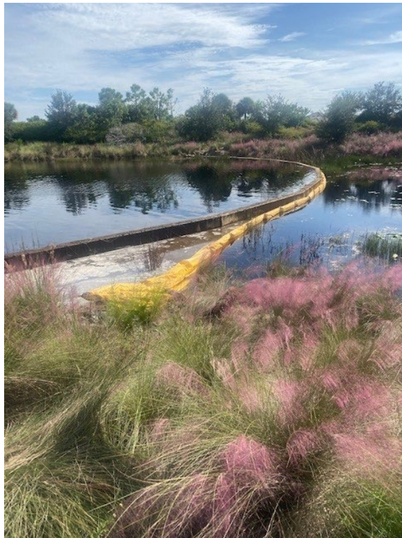
SWM - Flow Way Weir (South)
